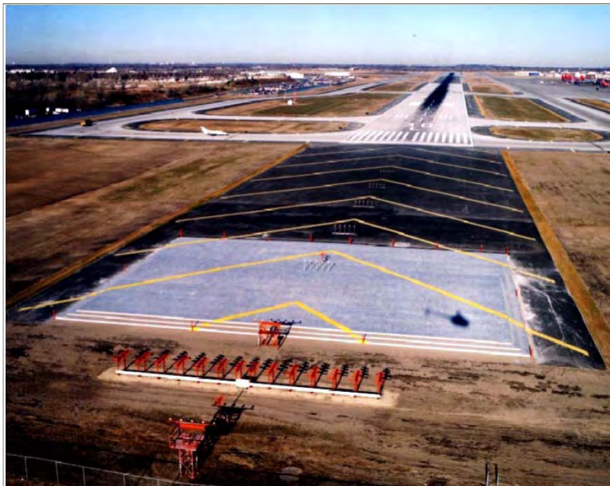
FIG 2-3-42 Engineered Materials Arresting System (EMAS)
